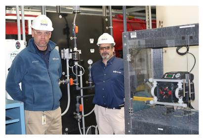
The hybrid CHEM-FEED MD3 diaphragm-type dosing pump has an excellent turndown ratio of 2000:1, and the gentle pumping action means no pulsation dampener is required. With 380 strokes per minute, the CHEM-FEED® MD3 provides a remarkably even, steady flow.
