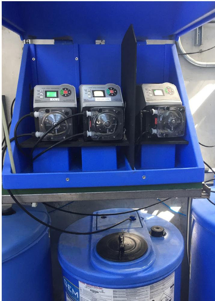
Two of the A2 pumps inject a solution of 12.5% sodium hypochlorite for use in the membrane bioreactor (MBR) filter backwashes. MBR processes can produce effluent of high quality so that it can be discharged into coastal waterways or be reclaimed for urban irrigation.
