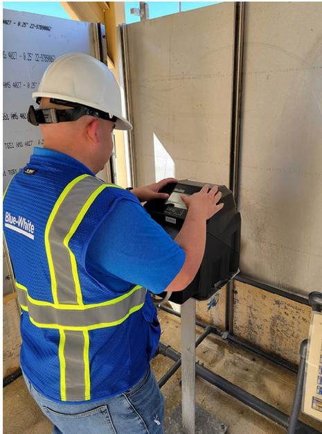
Figure 1. FLEXFLO® Peristaltic Pump Being Programmed at a WWTP.
